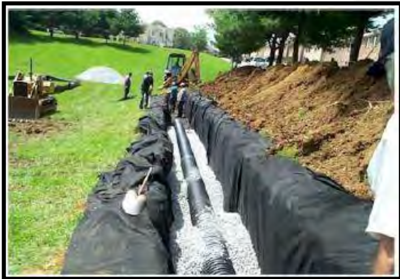
Photo courtesy of PADEP Stormwater Manual 2006
