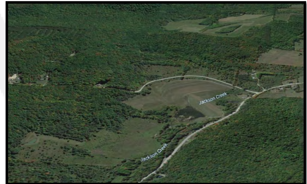
NY-5A Dam – Photo courtesy of Google Earth 2020
