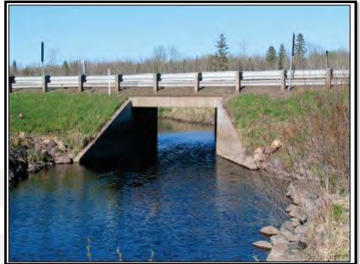
Photo courtesy of FHWA Hydraulic Design of Highway Culverts
