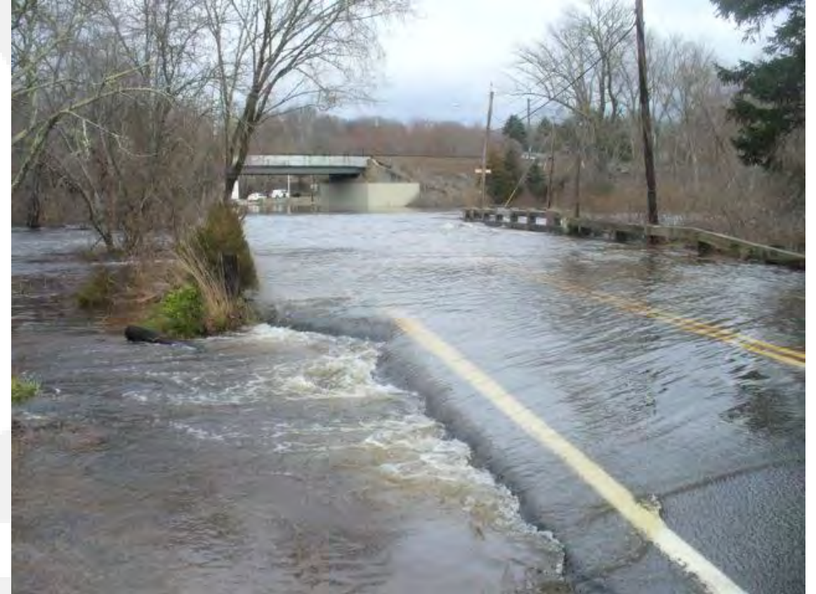
Shannock Road, Charlestown RI – March 2010
